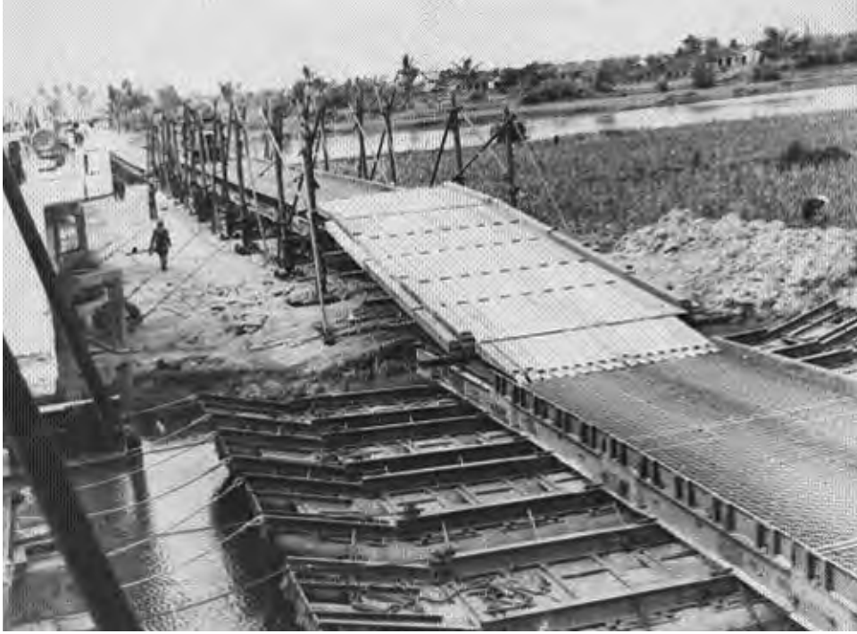
During Operation JOHN PAUL JONES, men of the 39th Engineer Battalion built a conglomerate bridge made up of several different tactical bridges.
